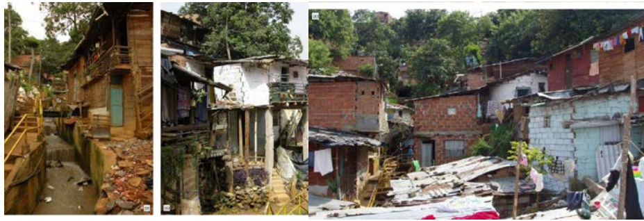
Figure 27: Conditions before PUI project upgrades
