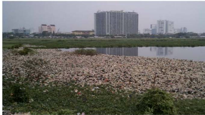
Figure 39: Water edge condition in Waduk Pluit
