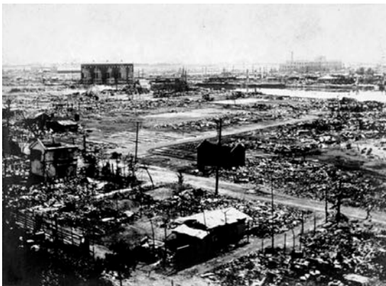
Figure 16: Kanto earthquake aftermath
