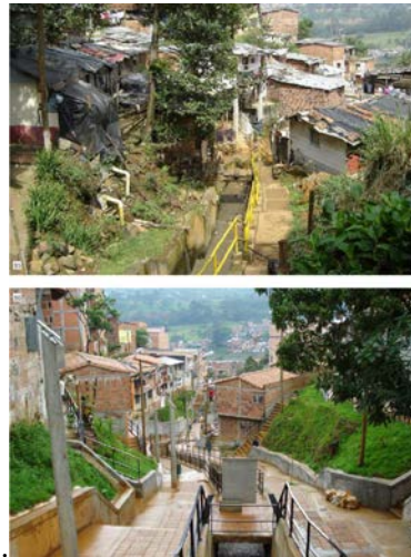
Figure 32: PUI circulation, runoff, and green infrastructure upgrade
